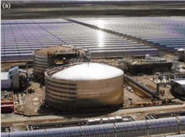
Figure 9 (a) Molten salt TES in Andasol Solar Power Station; (b) the system layout (daytime operation) [28].
